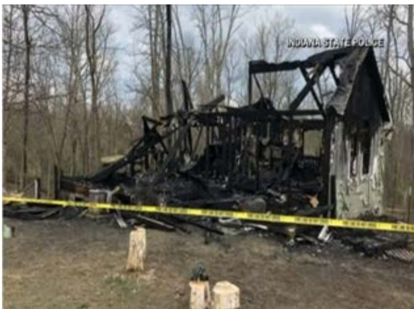
Figure 33 House Fire March 29, 2020, near Vevay
